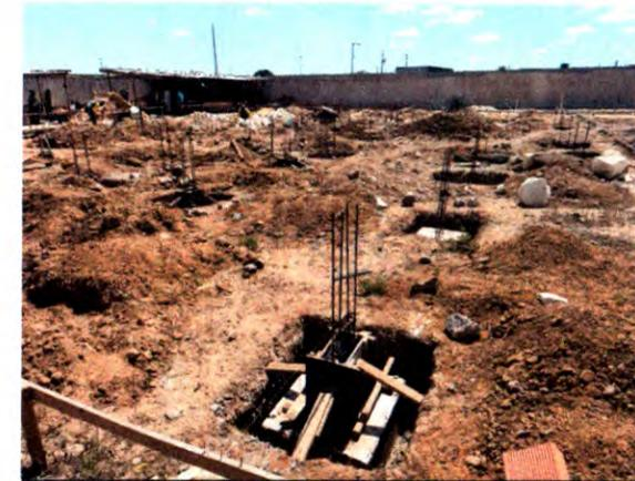
MONTAGEM DOS ARRANQUES E SAPATAS
