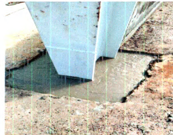
CONCRETO-EASE DOS PILARES
