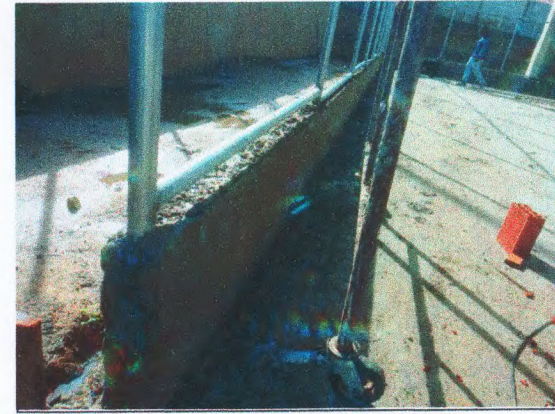
CONCRETO SIMPLES; ALAMBRADO
