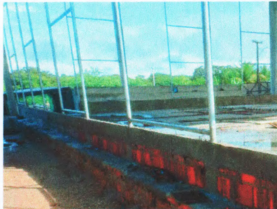
CONCRETO SIMPLES; ALAMBRADO;
