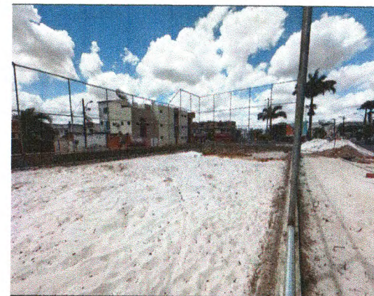
ALAMBRADO, ATERRO E REBOCO
