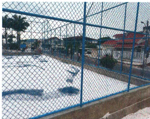
ALAMBRADO, ATERRO E REBOCO
